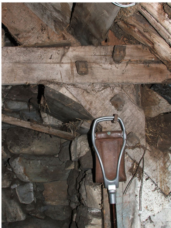
Figure 3. Inverey composite cruck-frame detail (photo: Coralie Mills)
