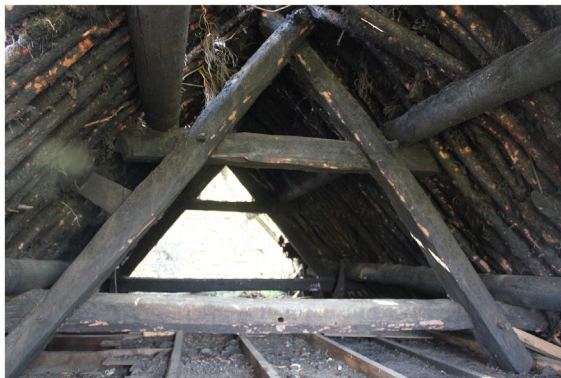
Figure 12b. Rooftruss at Badden Cottage, roof cabers (poles) also of pine (photo: Coralie Mills)
