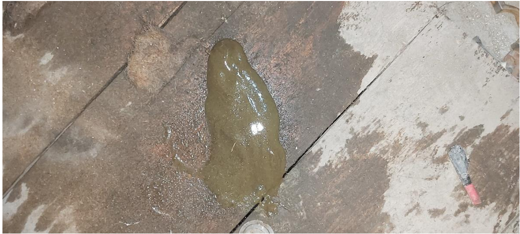
Figure 2 Biofilm (biological growth) from a length of dead leg removed from St Salvators' Hall by Estates Trades Nov 2020 – the amount of biofilm shown is sufficient to seed a whole system
