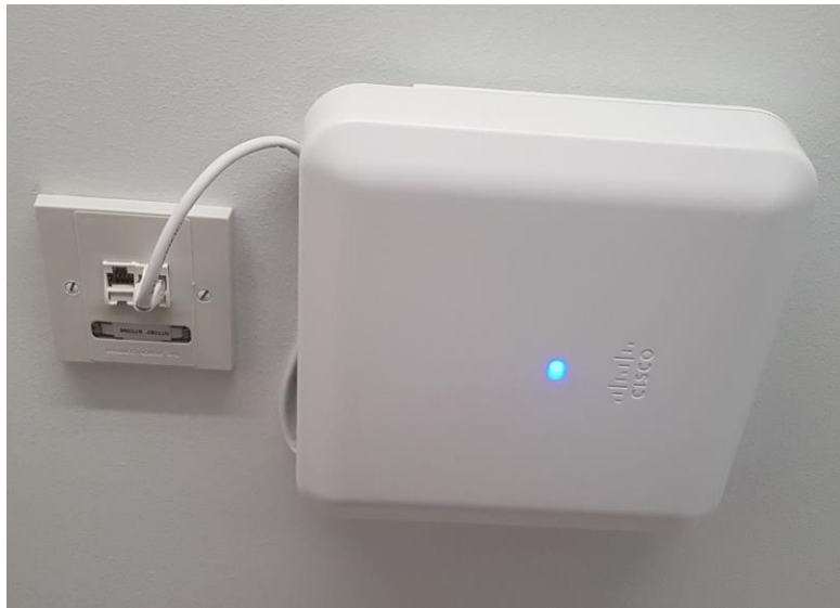
Figure 15.10:1 AP installation on solid ceiling
