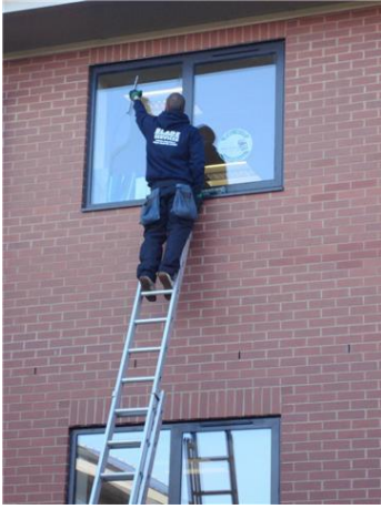
Access by ladder - Work at height
