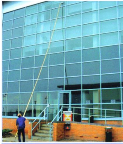
No work at height
