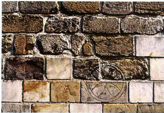
The West side of the tower shows the use of both older rough Nydie sandstone and newer Cullaloe stone. A consecration mark is clearly visible spanning both types of stone.
